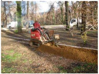
The ditch witch ploughed through the earth like a hot knife through butter, preparing trenches for new power cables to service future buildings. Not something you would want to do by hand, however, in some places large tree roots needed some elbow grease. Not an easy task working in tight places.
